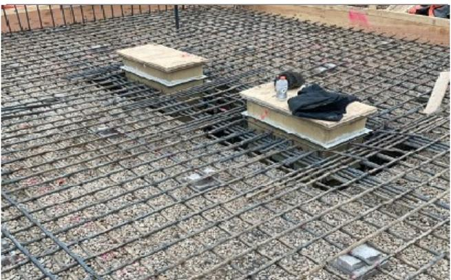
Floor rebar being installed around pool drains in deep section
