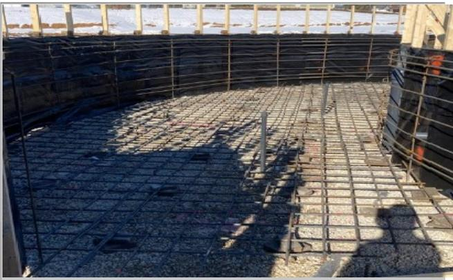
Rebar being installed for the North end of the river section
