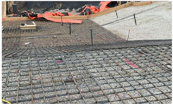
Floor rebar being installed in lap section of pool
