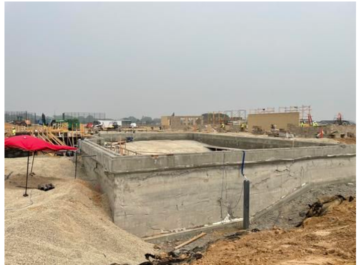
Lap pool and Bath house Masonry
