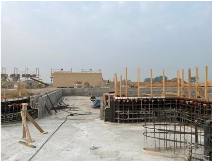
Leisure pool and masonry walls
