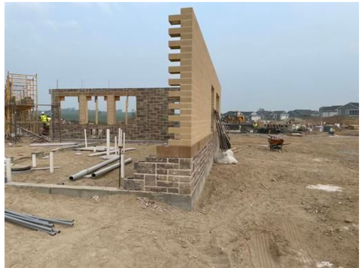
Masonry walls installed Bath House
