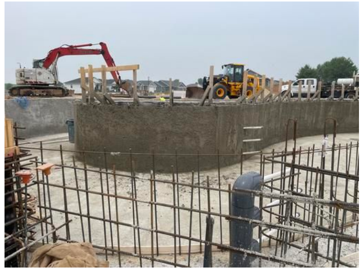
Lazy River walls poured
