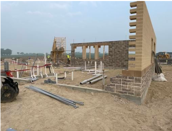
Masonry wall installation Bath House
