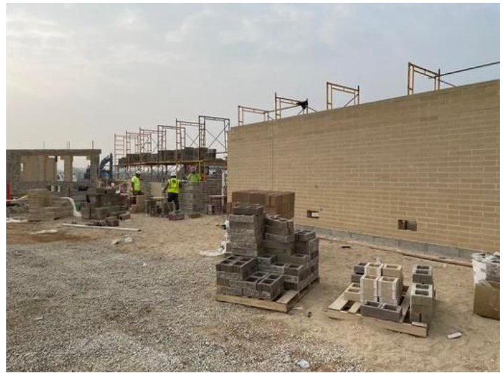
Bath House masonry wall installation
