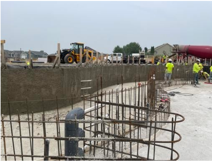
Lazy River walls poured
