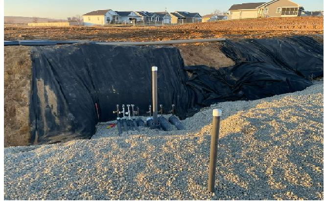
Deep pipes installed with pressure test on all pipes
