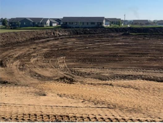
Baseball field topsoil stripped and read for fill
