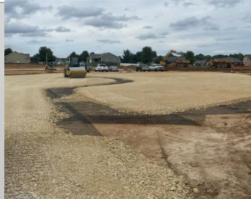
Parking lot 3" base stone being installed and compacted over geo-grid
