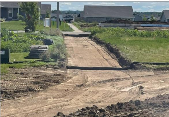
Sidewalk heading out to Porter Ave. cut to subgrade and compacted
