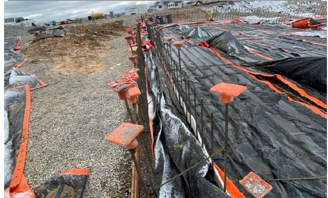
Lap pool floor covered for the weekend and wall rebar install beginning
