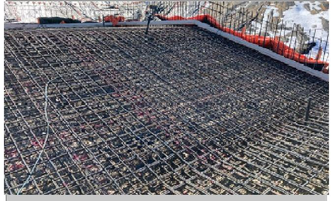
Rebar installed in lap pool floor, looking @ slope from shallow to deep end
