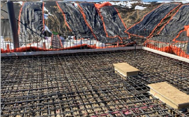
Rebar fully installed in lap pool floor
