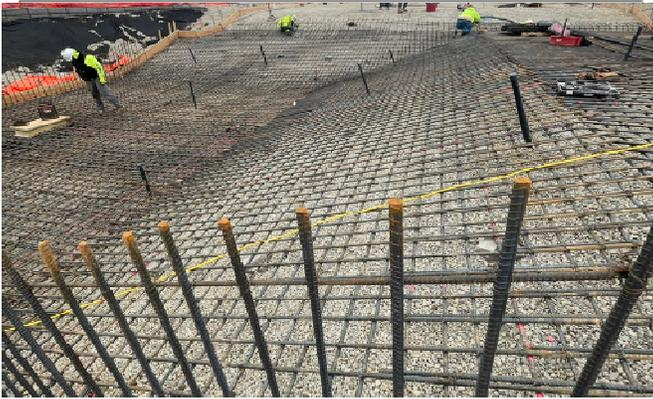
Rebar install @ lap portion of pool floor
