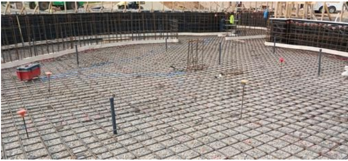
Lazy River floor rebar
