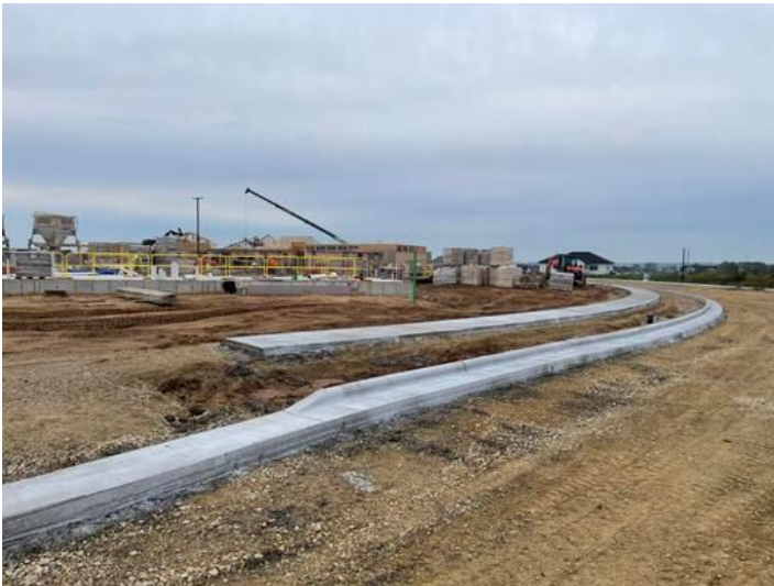
Installation of sidewalk and curb and gutter.
