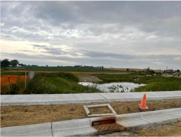
Installation of Sidewalk and Curb
