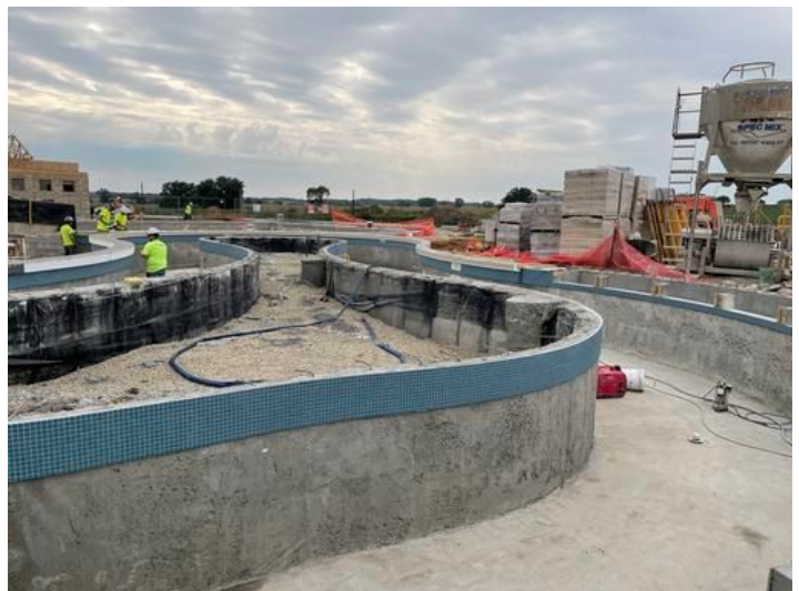
Lazy River Pool finishes Added on Sep 22, 2023, 9:36 AM CDT Added by andrew gordon
