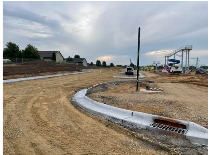
Installation of curb and gutter.
