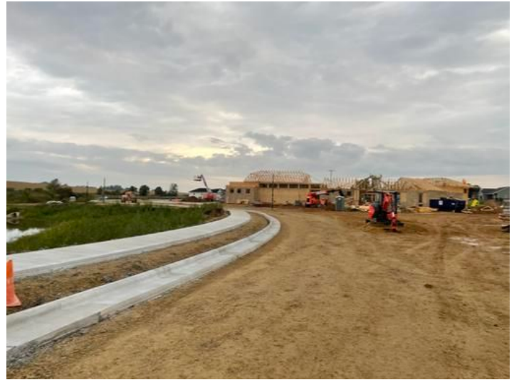
Installation of Roof trusses
