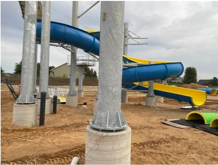
Installation of Waterslide
