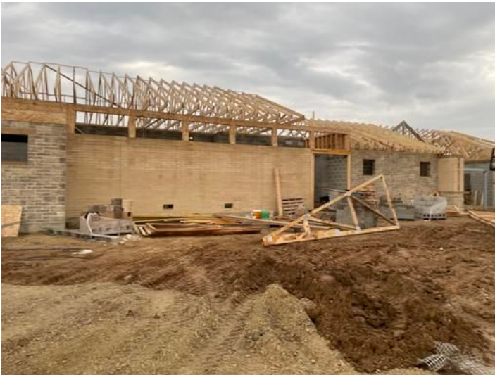
Installation of Roof Trusses.
