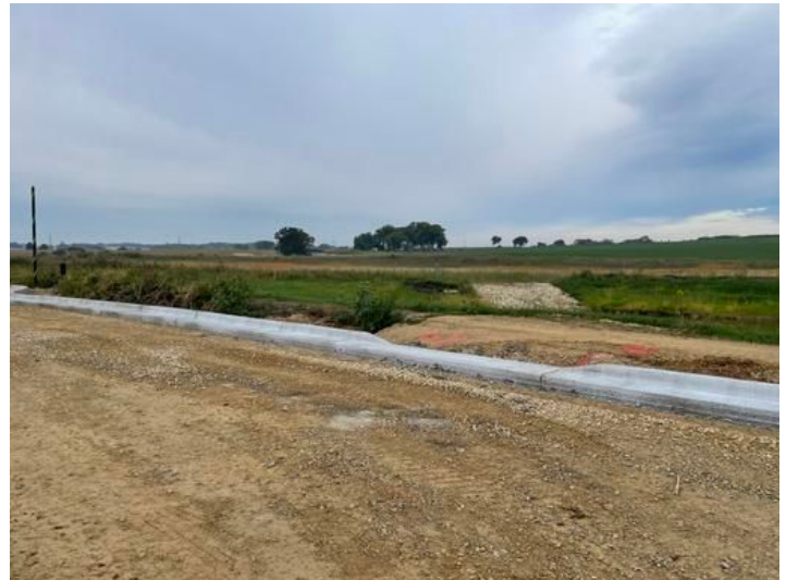
Installation of curb
