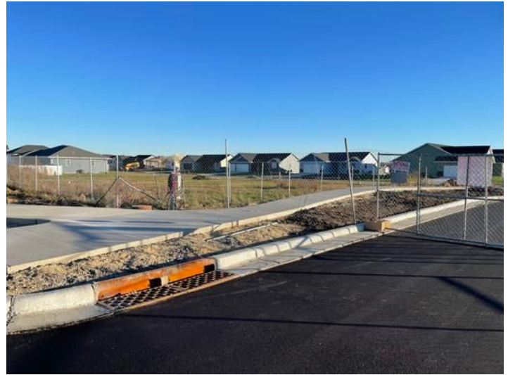
installation of Sidewalks
