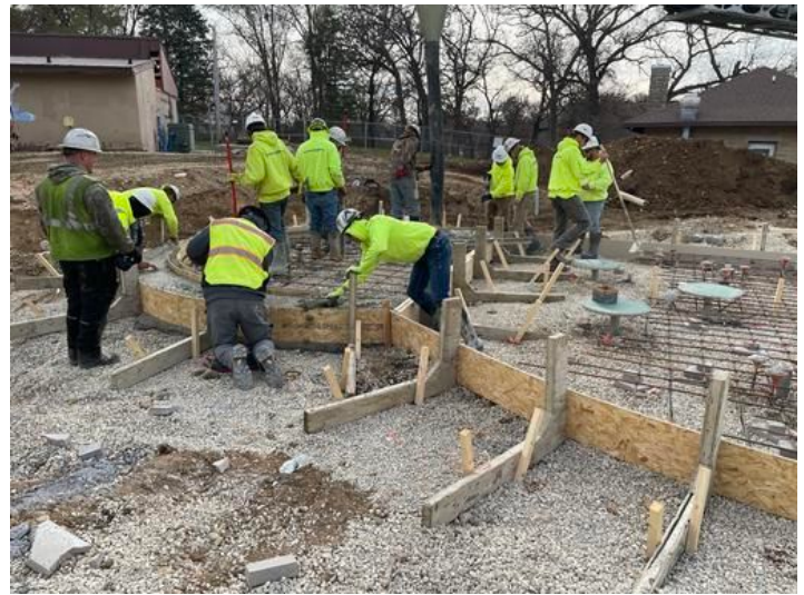
Installation of Splash Pad concrete Taken on Nov 16, 2023, 10:16 AM CST Added on Nov 16, 2023, 12:29 PM CST Added by andrew gordon
