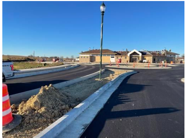
ready for Top soil.
