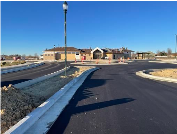
Installation of curbs
