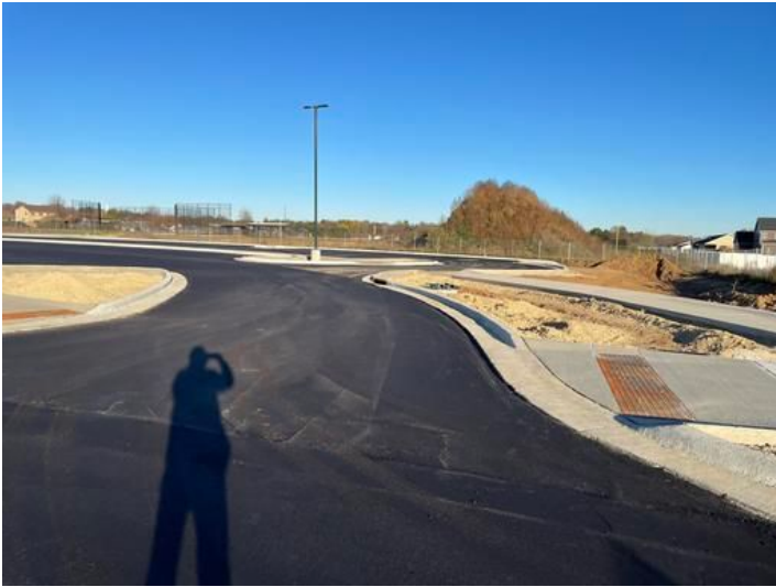
Installation of Sidewalks.
