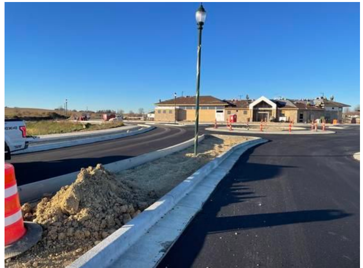
ready for Top soil.
