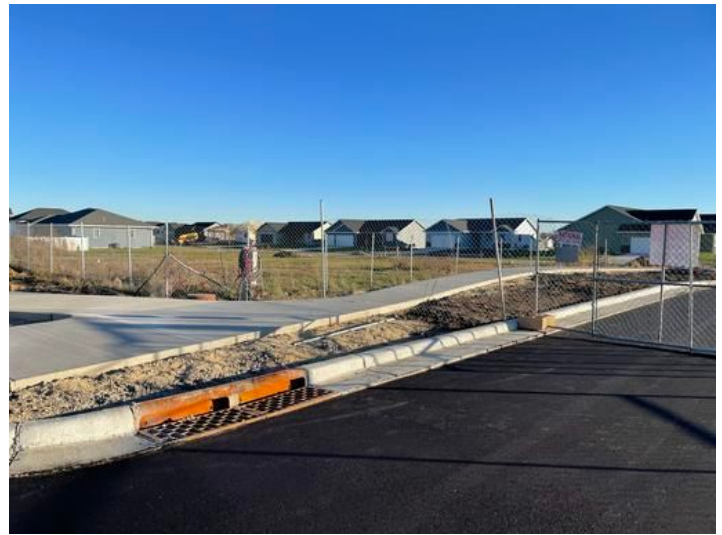
installation of Sidewalks
