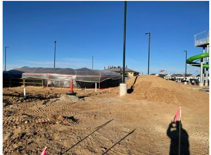
Installation of Tile for Lazy River Pool entry enclosure.
