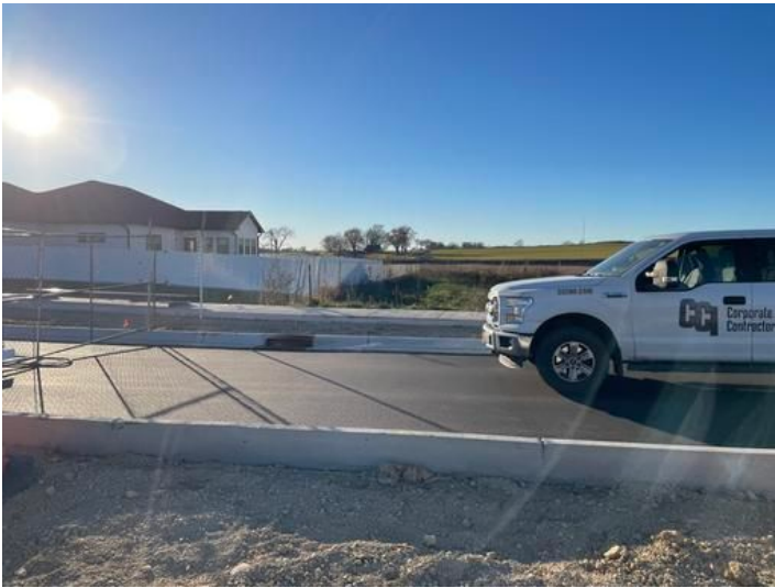
Installation of Binder
