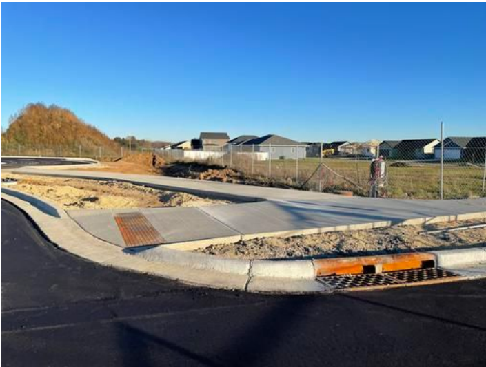
Installation of Curb and Sidewalks.
