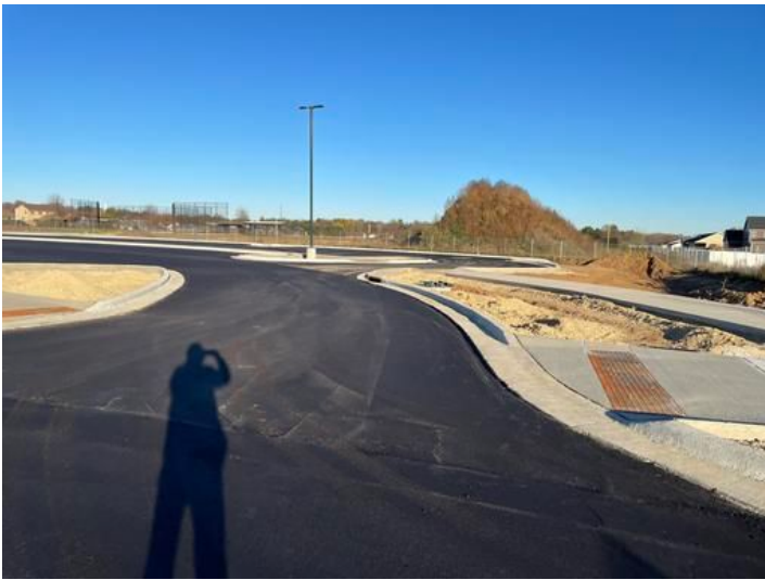
Installation of Sidewalks.
