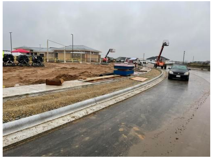
Sunshades installed Taken on Nov 8, 2023, 9:28 AM CST Added on Nov 8, 2023, 10:15 AM CST Added by andrew gordon
