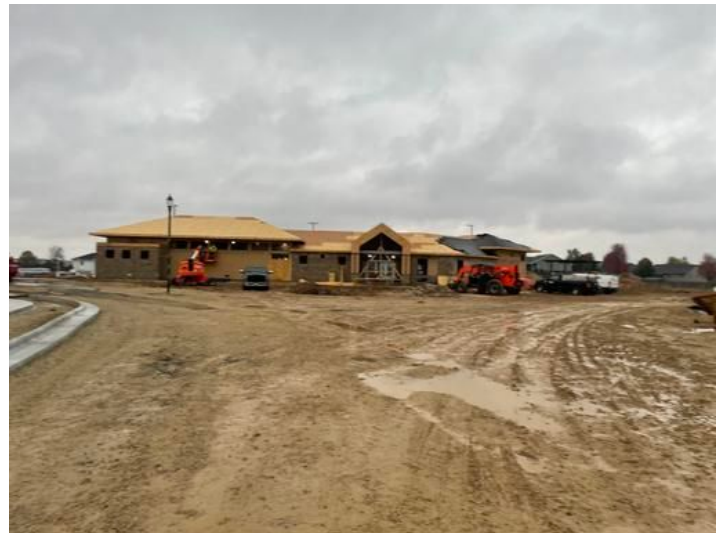
Site Work to start on south and East side.
