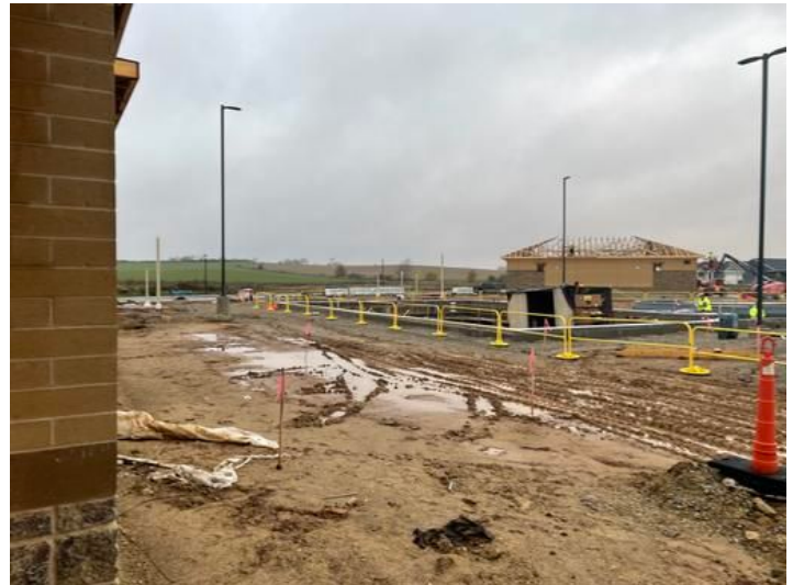
Stake out for Deck Drains.
