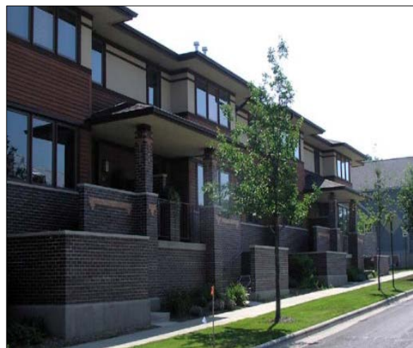
FIGURE10F: PRAIRIE STYLE TOWNHOMES RESPECT REGIONAL ARCHITECTURE IN MIDDLETON HILLS, A TND IN MIDDLETON, WI. Image Source: dkolb.org
