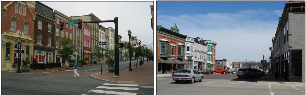
FIGURE 10X: THE HIGHLY RATED IMAGE FROM THE 2015 VISUAL PREFERENCE SURVEY (LEFT) PROVIDES EXAMPLES OF FURTHER STREETScape, SUCH AS CURB EXTENSIONS, THAT COULD ENHANCE EVANSVILLE'S DOWNTOWN (RIGHT).
