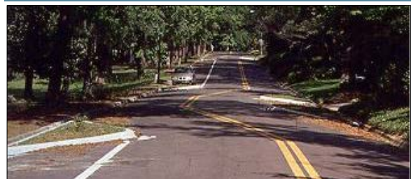
Chicanes are curb extensions that extend from one side of a street to the other forming s-shaped curves.
