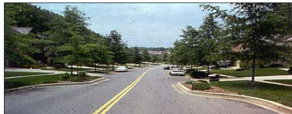
Chokers – Used to Narrow Street width and slow traffic. Can accommodate on-street parking. Potential for use along W. Main Street, 5th and 6th Streets.
