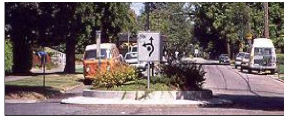
Traffic Circle – A circular arrangement constructed at intersections of two or more roads.
