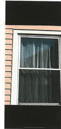
Dining Room Window @ side of House
