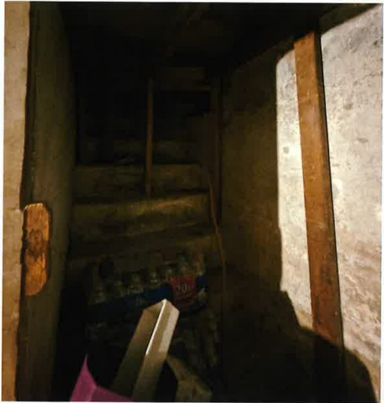
Abandoned original stairs.
