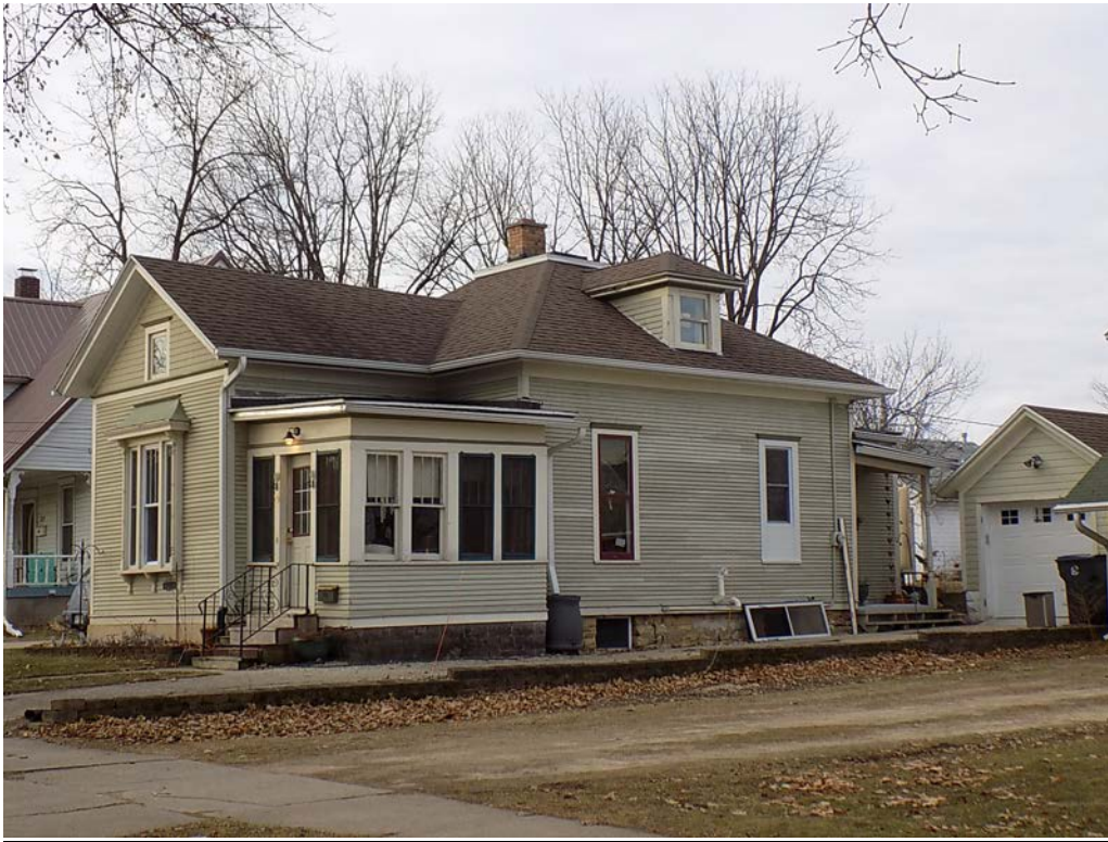
HPC-2019-68 , Site Photos Taken Dec 2019
