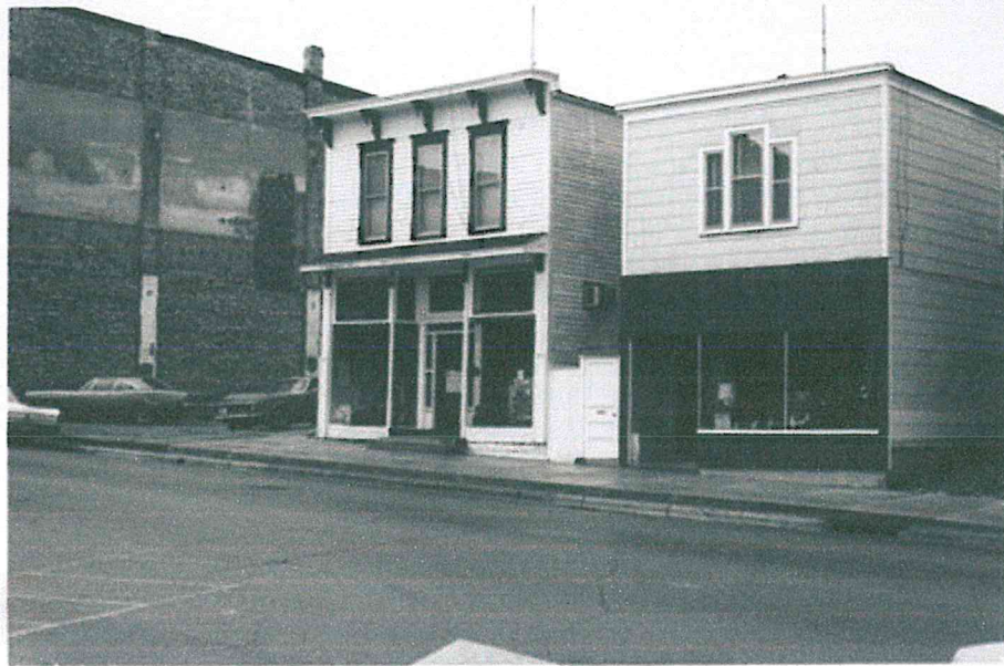
Rock Co. EVANSVILLE 008 5235 (left); 008 5277 (right) 24-26 E. Main
