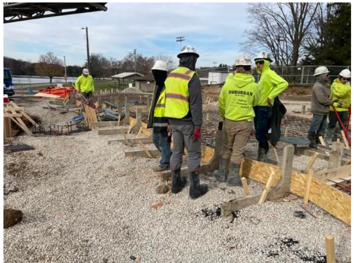
Prepare for Splash Pad concrete pour. Taken on Nov 16, 2023, 10:12 AM CST Added on Nov 16, 2023, 12:24 PM CST Added by andrew gordon
