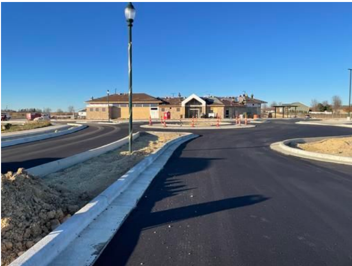
Installation of curbs
