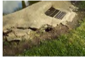
Allen's Creek Rip-Rap at East L
