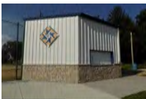
North Baseball Diamond Building
