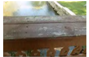
510 Allen's Creek Footbridge
