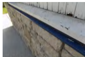
North Baseball Diamond Building
