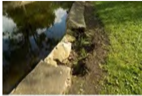
Allen's Creek Rip-Rap at East L
