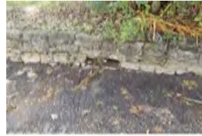
1426 Retaining Wall near Public Works Building
