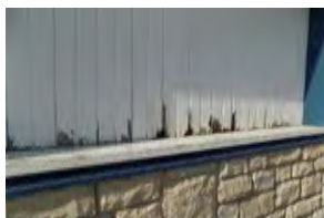
North Baseball Diamond Building
