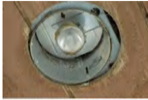
512 Allen's Creek Footbridge
