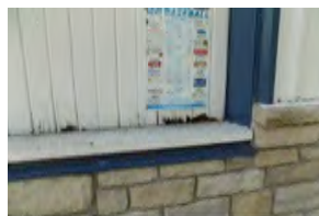
North Baseball Diamond Building
