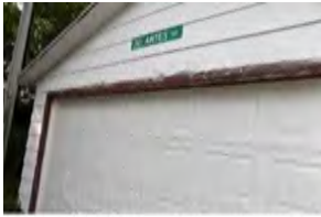
1418 Department of Public Works Building
