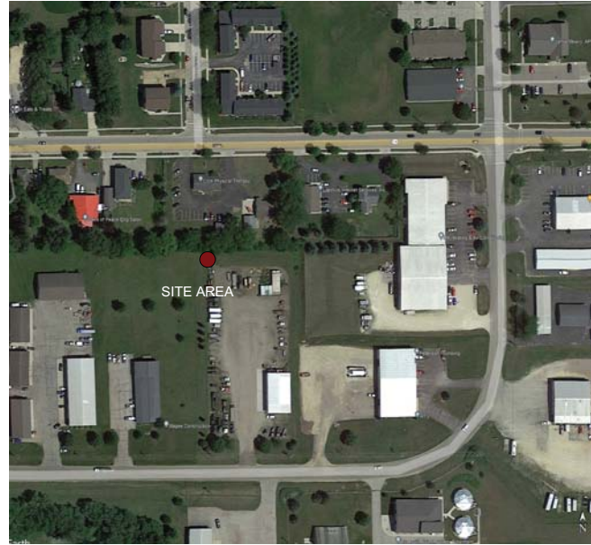
AERIAL VIEW OF SITE
