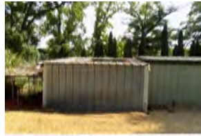
Department of Public Works Building
