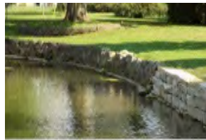
603 Allen's Creek Rip-Rap
