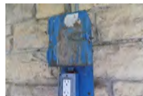
324 Henneberry Shelter House
