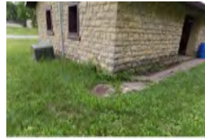
308 Henneberry Shelter House
