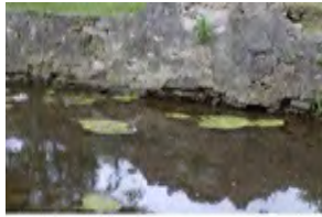
Creek Rip-Rap Horseshoe La
