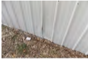
Department of Public Works Building
