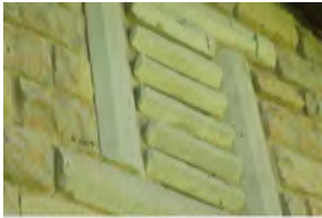
330 Henneberry Shelter House
