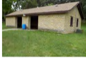
302 Henneberry Shelter House
