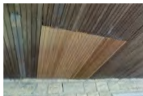
322 Henneberry Shelter House
