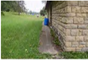
305 Henneberry Shelter House
