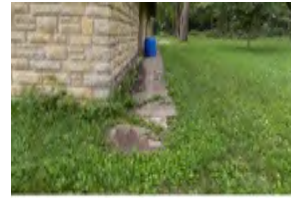
309 Henneberry Shelter House
