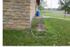
304 Henneberry Shelter House
