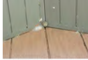
504 Allen's Creek Footbridge
