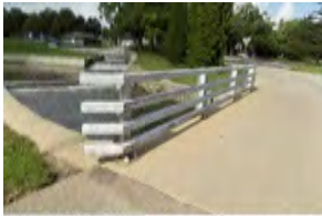
White Drive Bridge Over Allen's
