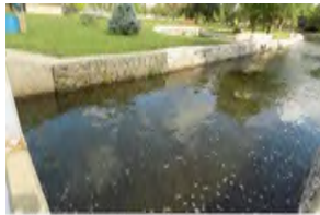
607 Allen's Creek Rip-Rap
