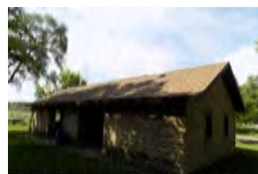
328 Henneberry Shelter House
