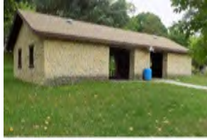
301 Henneberry Shelter House
