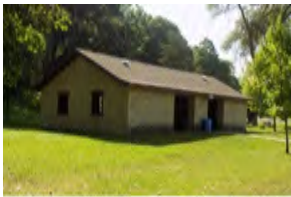
310 Henneberry Shelter House
