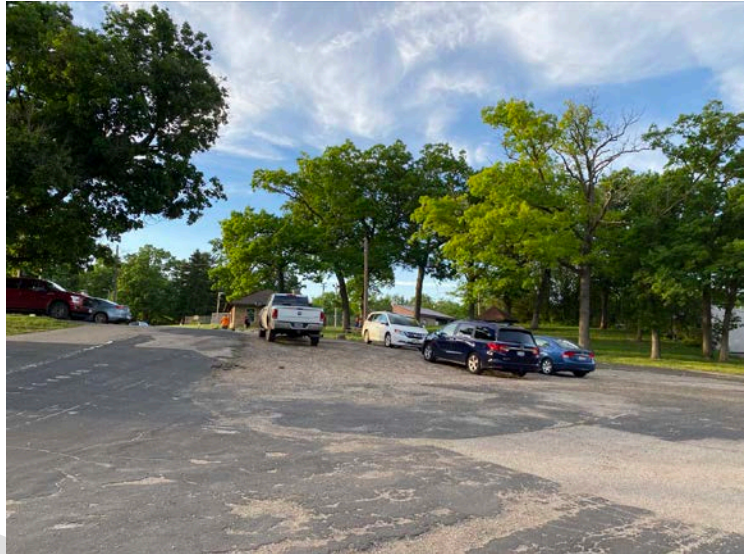
FIGURE 6.4 EXAMPLE OF ADDED PAVEMENT
