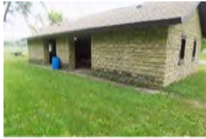
306 Henneberry Shelter House
