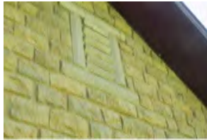
331 Henneberry Shelter House
