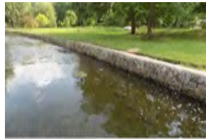
608 Allen's Creek Rip-Rap
