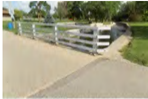
White Drive Bridge Over Allen's
