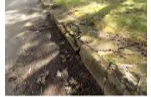
Retaining Wall near Public Works Building
