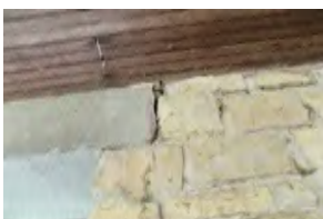
325 Henneberry Shelter House
