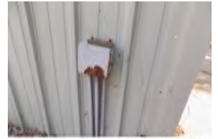
Department of Public Works Building
