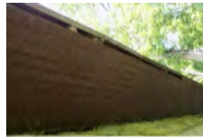
313 Henneberry Shelter House
