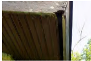
312 Henneberry Shelter House
