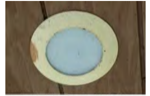
515 Allen's Creek Footbridge
