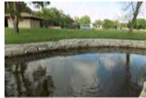
Creek Rip-Rap at Horseshoe L
