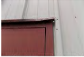
Department of Public Works Building
