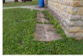
303 Henneberry Shelter House
