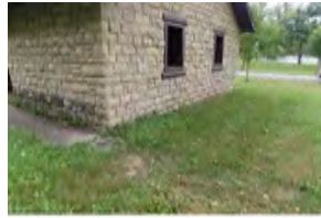
307 Henneberry Shelter House
