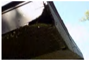
311 Henneberry Shelter House
