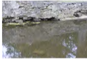
Creek Rip-Rap Horseshoe La
