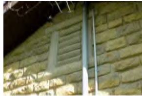
332 Henneberry Shelter House
