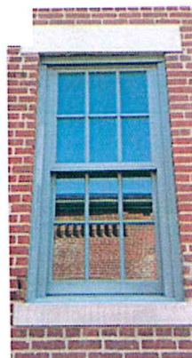
A replacement window should match the original in design, dimension and, where possible, materials. Here is an excellent example of a replacement window. Source: Bob Yapp
