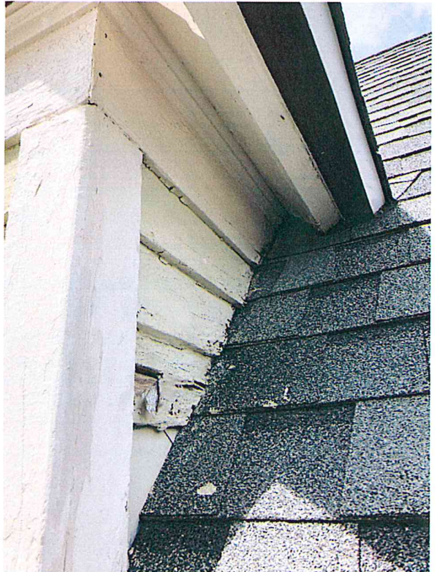
4. "RIGHT" SIDE OF DORMER
